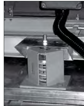
2.0" Seismic type spring isolator
